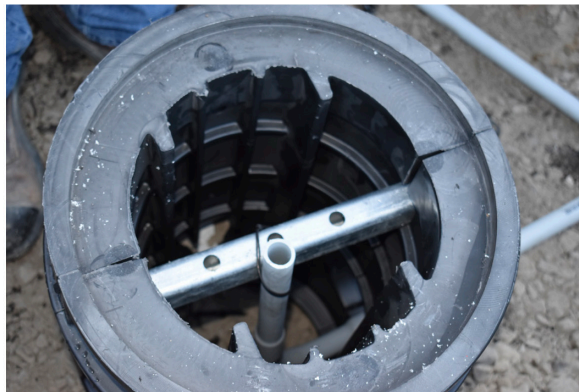
Conduit can be tie wrapped or wire tied to the middle bar for support.
